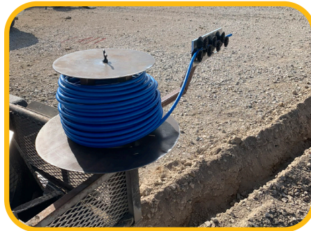
MaxLine spool and trench
