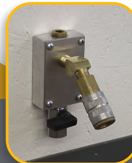
Hidden Mount Air line is inside wall
